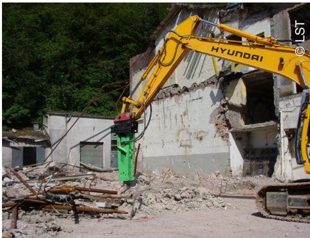
Hydraulic breaker GS 501 on a Hyundai 210 on the Romika site near Trier.
